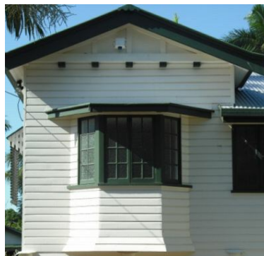
Figure SC6.2.3.16 Illustrates an example of projecting bay window with four casement frames two located centrally and one either side
