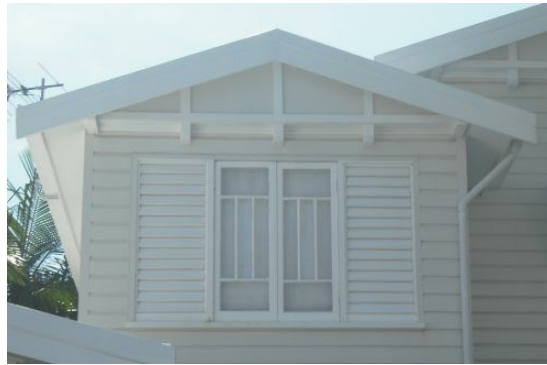
Figure SC6.2.3.14 Illustrates an example of two vertically proportioned casements and louvers either side, centrally located under the apex of a gable projection
